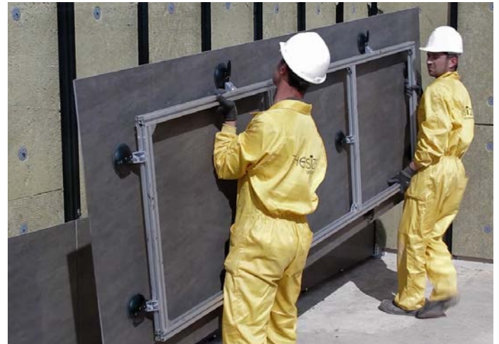
Image 7: Slab handling with Suction Frame
