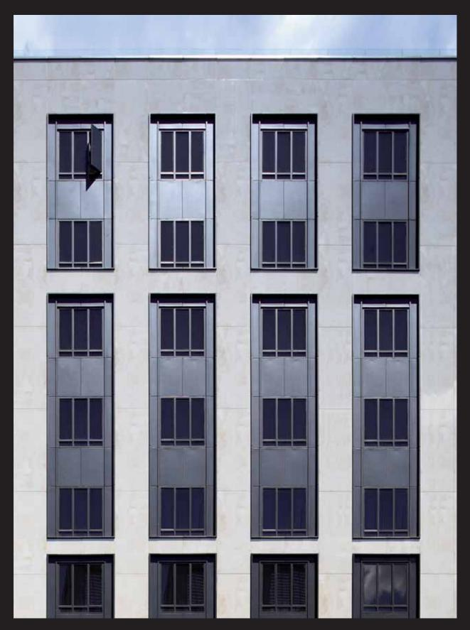
Ventilated Facade: **Onyx Polished, 6 mm** Cladding System: **HC System**
