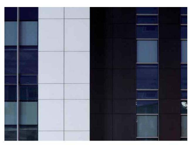
Ventilated Facade: **Basalt Black & Nieve, 6 mm⁺** Cladding System: **HC System**
