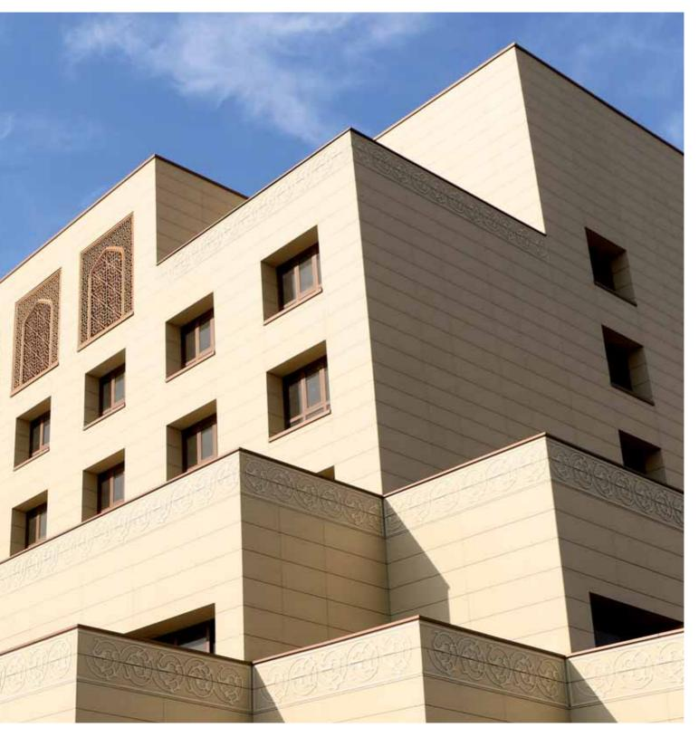
Ventilated Facade: **Basalt Beige, 6mm⁺** Cladding System: **VM System**
