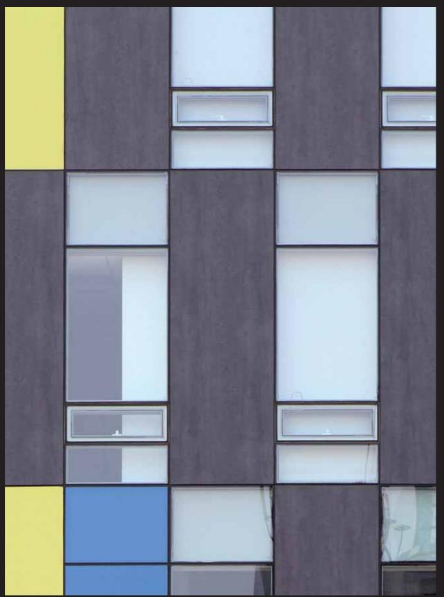
Ventilated Facade: **Basalt Black & Mela, 6 mm⁺** Cladding System: **HC System**
