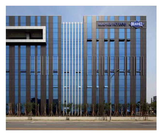
Ventilated Facade: Iron Grey 6, mm⁺ Cladding System: Curtain Wall
