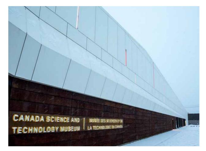
Ventilated Façade: Arctic White, 6 mm⁺ Cladding System: Ceramitex
