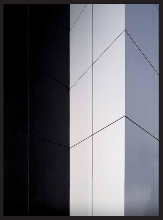
Ventilated Facade: **Basalt Black & Nieve, 6 mm**⁺ Cladding System: **HC System**
