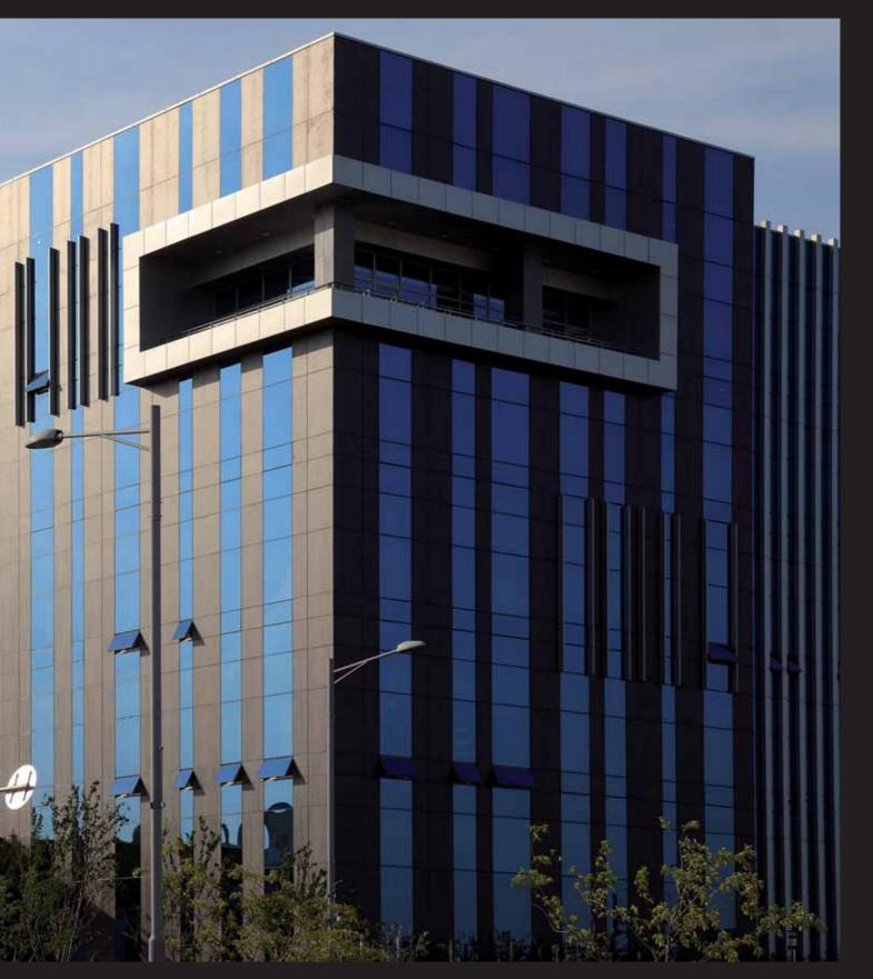
Ventilated Facade: **Iron Grey 6, mm⁺** Cladding System: **Curtain Wall**
