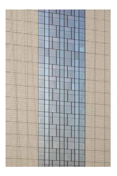
Ventilated Facade: **Arena, 6 mm⁺** Claading system: **Curtain Wall**
