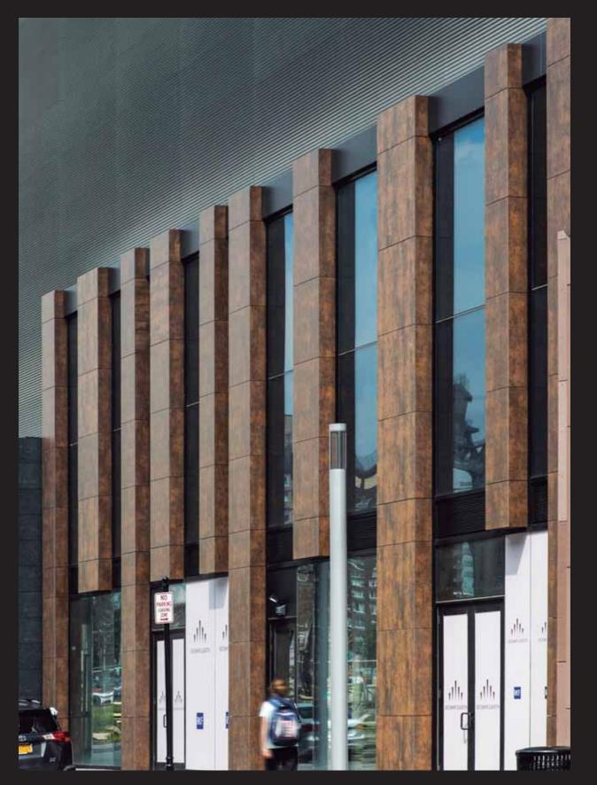
Ventilated Facade: Iron Corten & Pierre Bleue, 6 mm<sup>+</sup> Cladding System: Strongfix System
